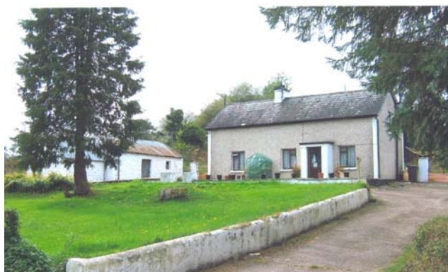
The former office at Drumcask - September 2007
