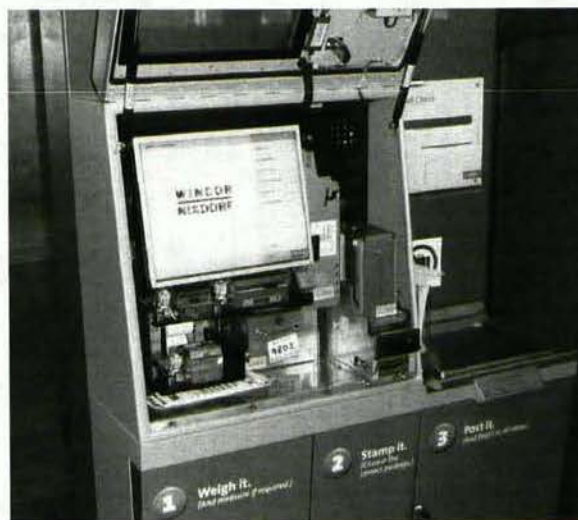
Dublin Airport machine with touchscreen in open position during repair work
